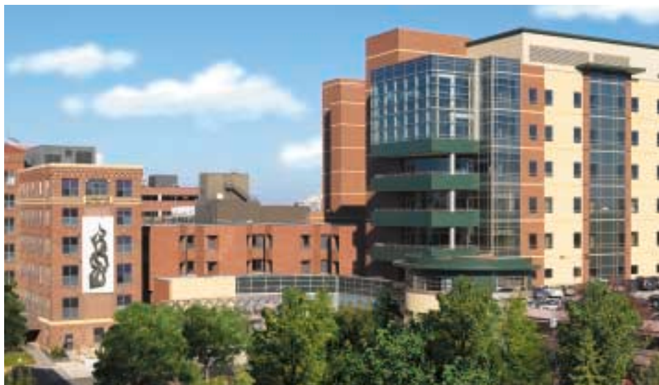
The Heart Hospital stands as a new landmark of heart care and consolidates all cardiology services into one building.
